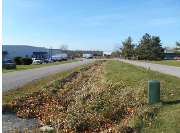
Figure 3: Industrial Park median swales, which drain to the area of the proposed new detention pond.
