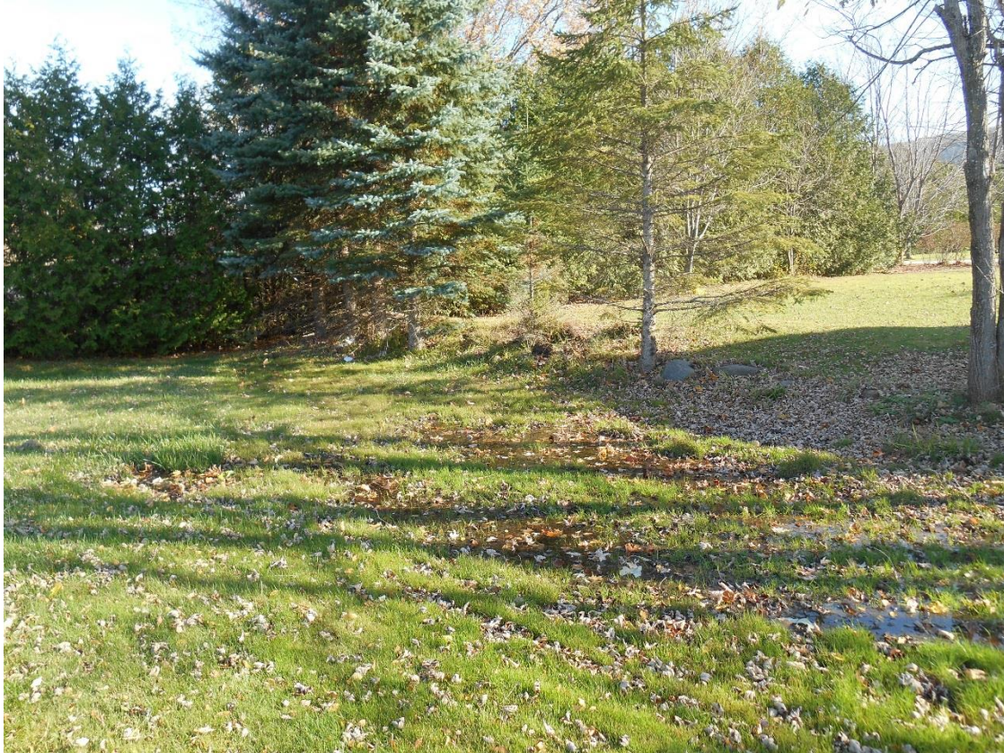
Figure 6: Low area between homes along Clyde Allen Dr. with history of flooding. New footing drain and outlet proposed to drain area.
