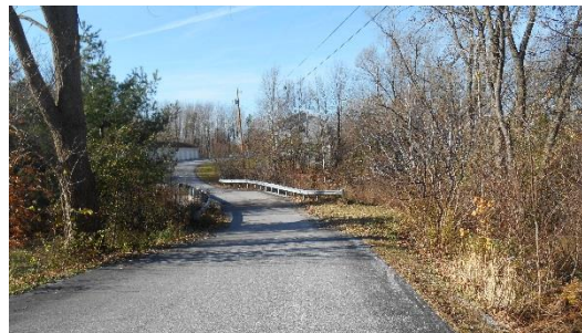
Figure 4: Rugg Brook crossing at end of Twin Court.
